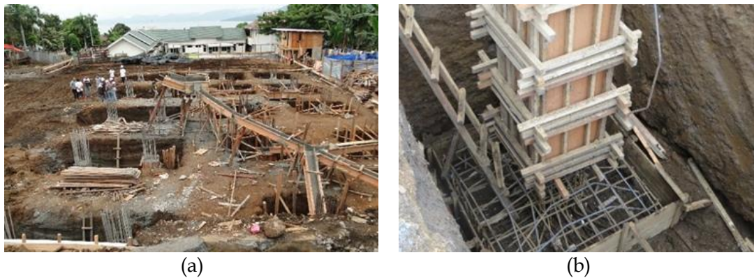
Figure 6. Foundation design structure after modification in this study; (a) Planned in design foundation, (b) Detailed reinforcement after modification
