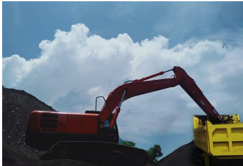
Gambar 7. Dumping Material Hitachi ZX 200
