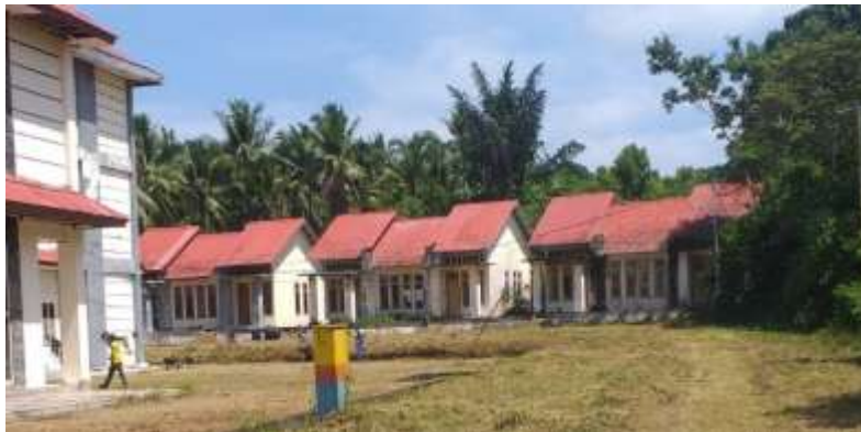
Figure 3. Lecturer's House Campus 4 Sofifi
