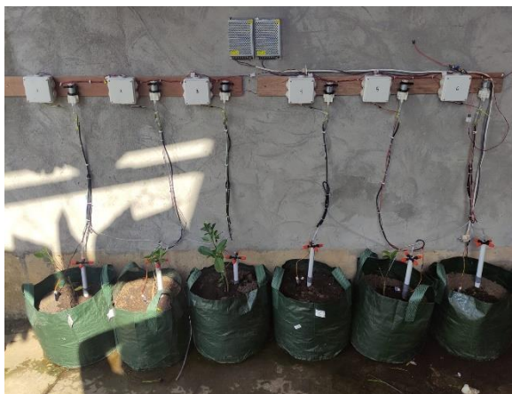
Figure 9. Installation of the System on Potted Fruit Plants
