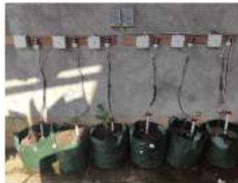
Figure 8. Installation of the System on Potted Fruit Plants
