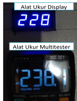
Figure 13. Inverter Output Voltage
