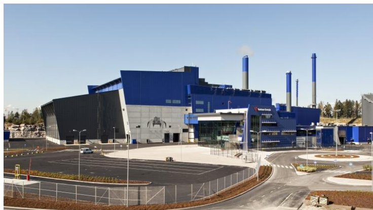
Gambar 5. Incinerator Waste to Energy di Helsinki-Finlandia [59].
